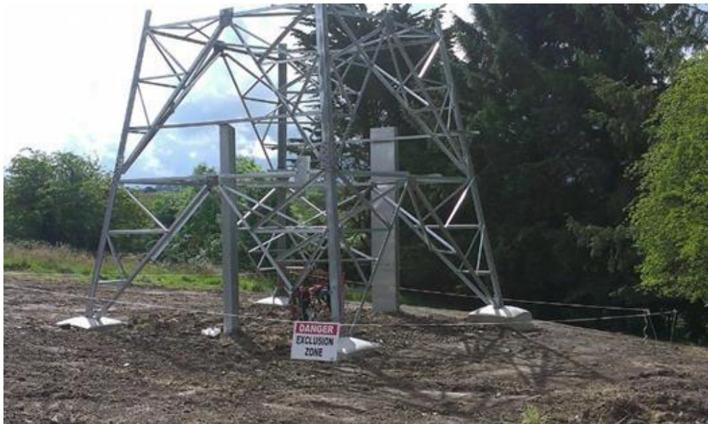
Plate 2.3: Base of an interface mast structure backfilled
