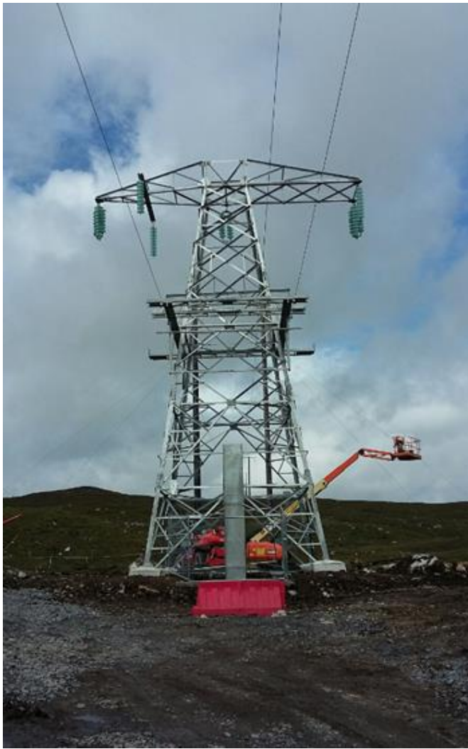
Plate 2.4: A completed line/cable interface mast
