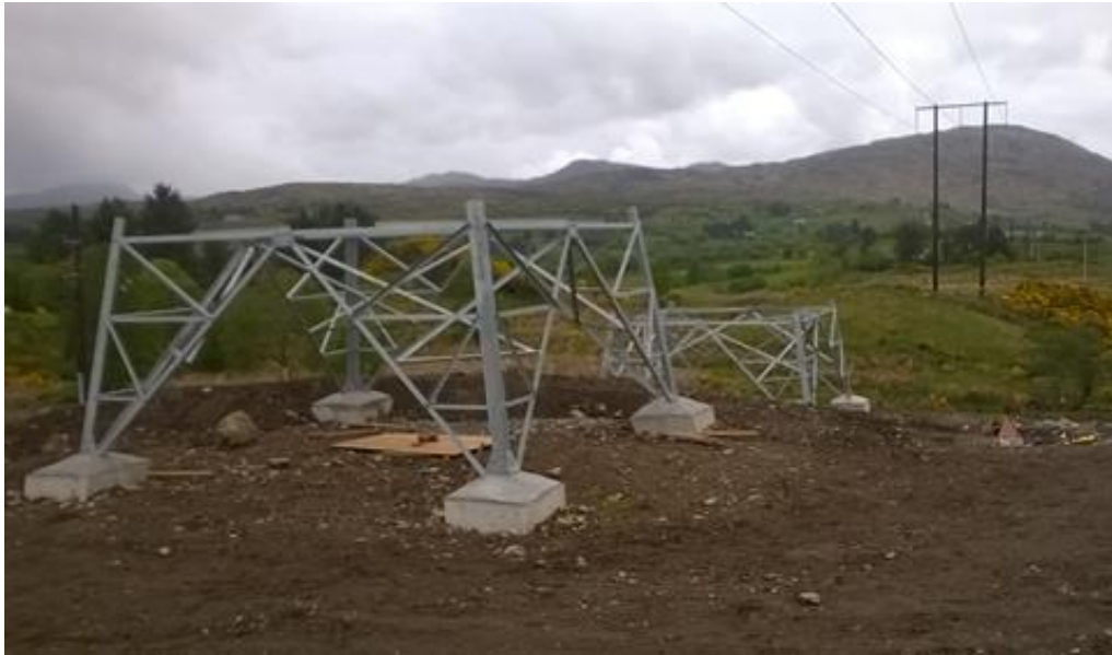
Plate 2.2: A 110 kV interface mast foundation complete
